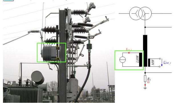
Figure 24: Spare power auxiliary winding (PAW) for current injection
